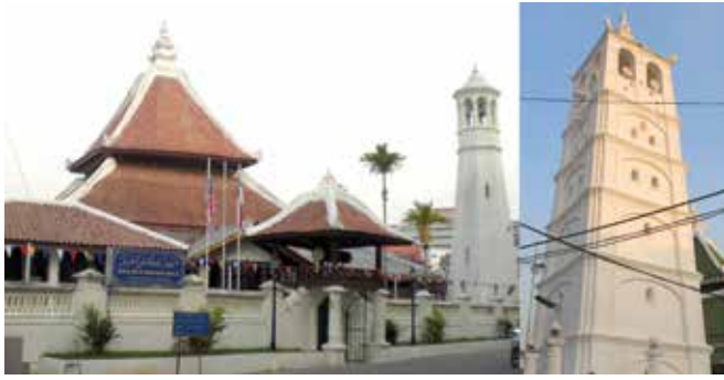
Fig 5 Roof finials (memolo) and roof ridge-end ornaments (sulur bayung) on mosques and minarets in Melaka: Kg Hulu (left) and Kg Keling Mosque, photos by the author
